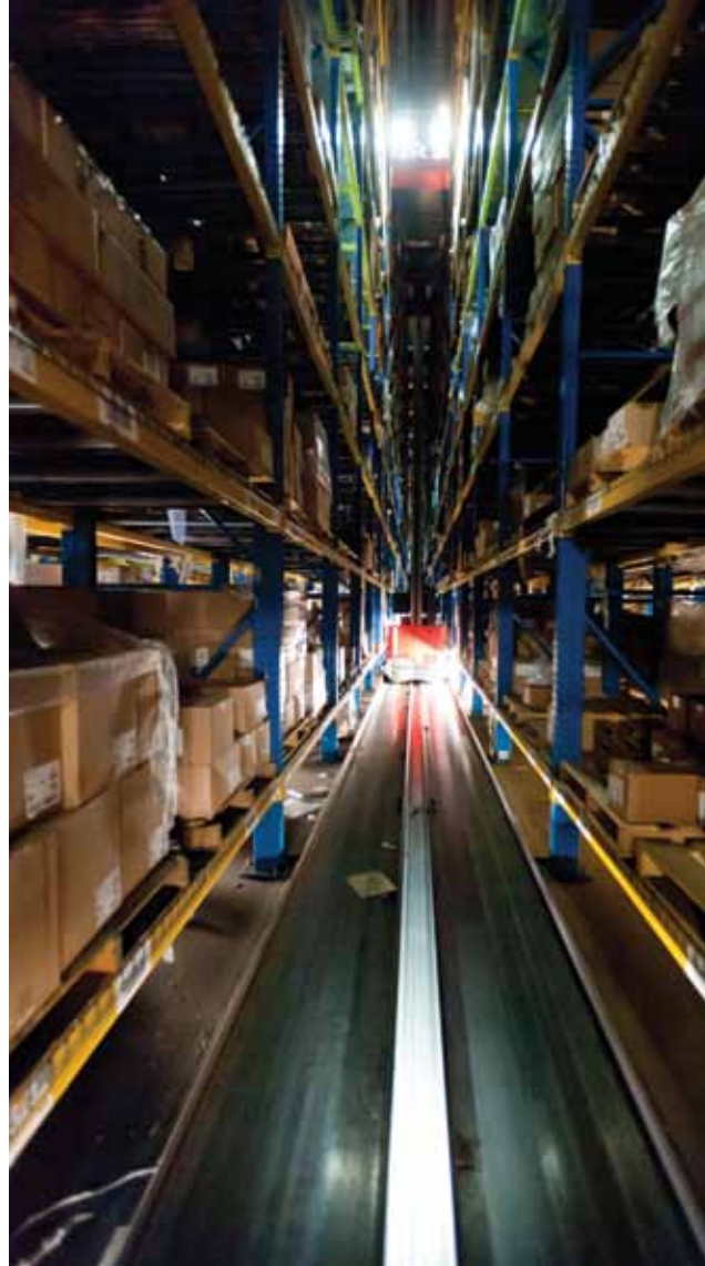
Narrow-aisle wire-guided turret trucks are used for putaway and picking in the full-pallet storage area.
